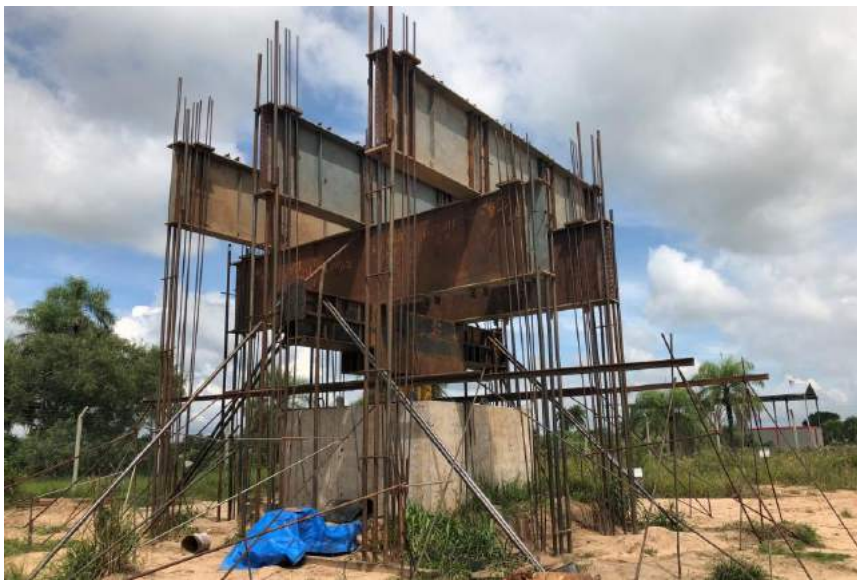
Fig. 9 Photo of set-up for head-down test on the E-Group.
